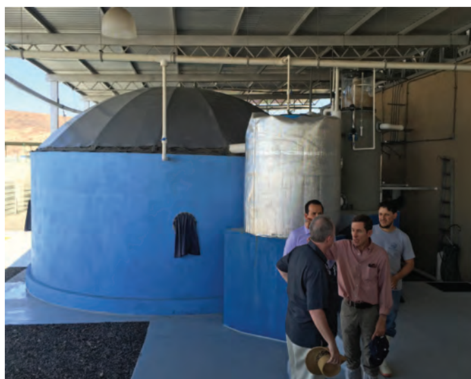
FIGURE 6. One of Earth Ocean Farm’s 80-m 3 totoaba broodstock maturation tanks. Note cover to allow photoperiod manipulation, windows to observe fish behavior, and water recirculation equipment on the right. EOF photo by Lorenzo Juarez.
