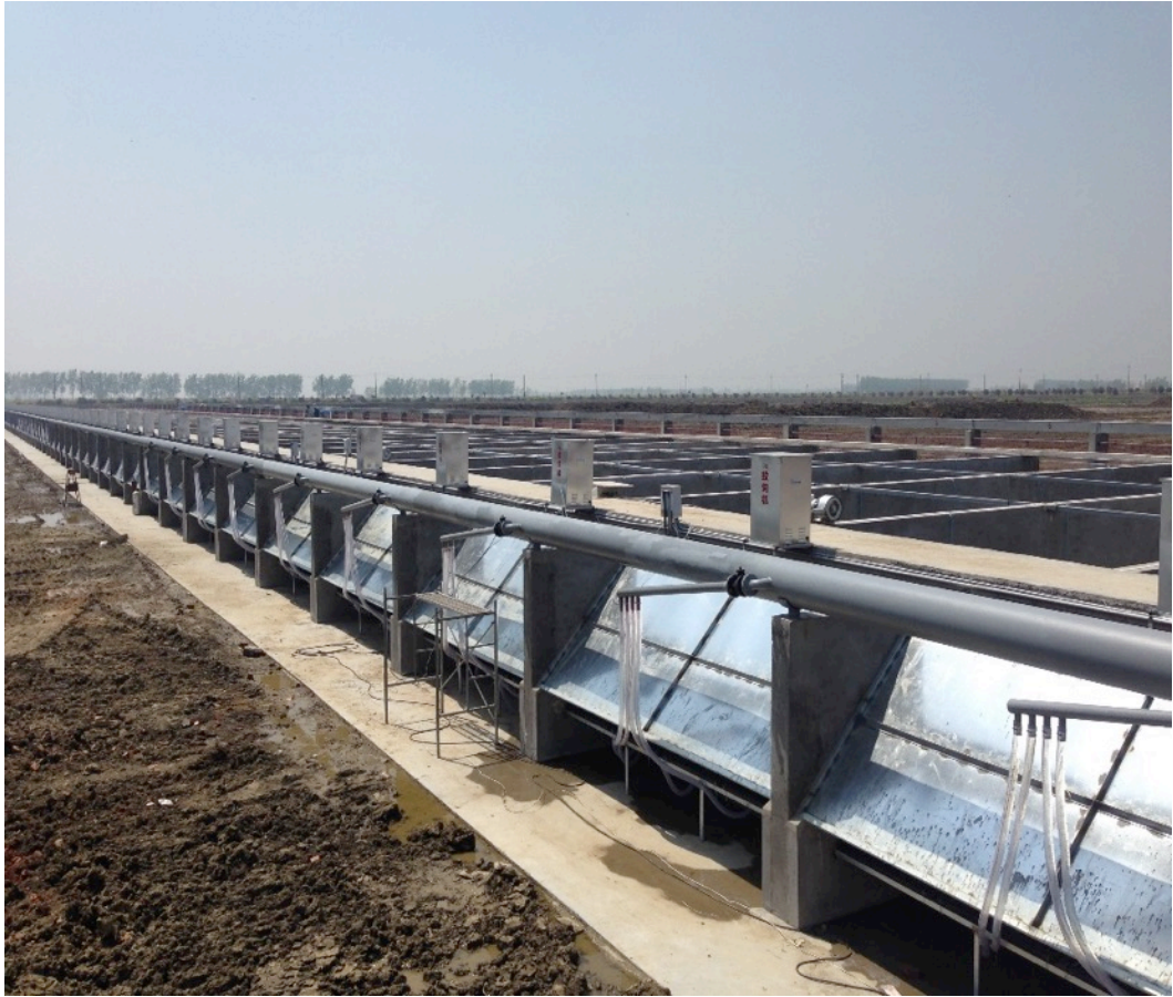
Front view of 52-cell IPA unit before water gets in
