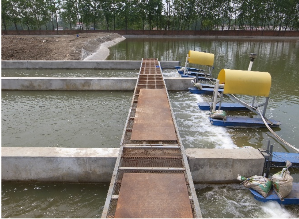
The water-pushing appliances in front of the IPA raceways
