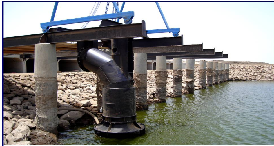
Installing The First of ten Pumps
