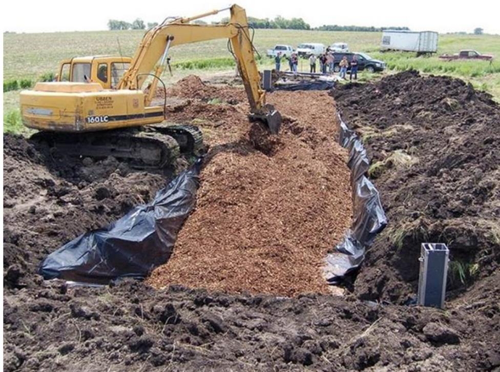
Woodchip denitrification bioreactors are an increasingly common “in-field” N-mitigation technique. Installation consists of a large lined trench filled with woodchips that water is routed through. Once installed they may be covered with soil and grass. Photo by L. Christianson/Iowa Soybean Association Environmental Programs and Services.
