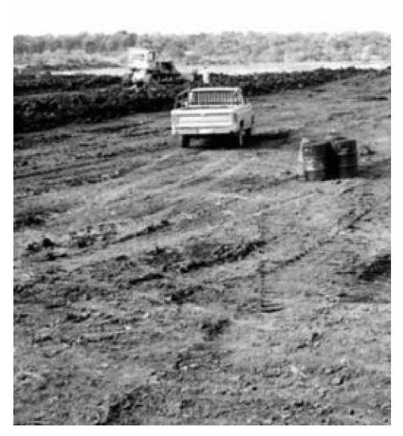
Embankment ponds are made by digging soil from the bottom to build up levees.
