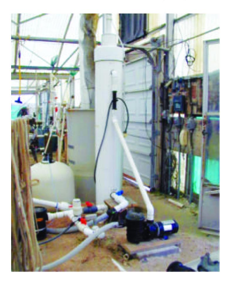
The large size of the foam fractionators allowed them to quickly reduce particulate loads but made precise control of solids levels a challenge.
