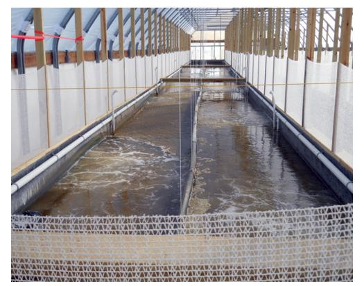
This 100-m<sup>3</sup> biofloc raceway is operating with an injector system that reduces oxygen use.
