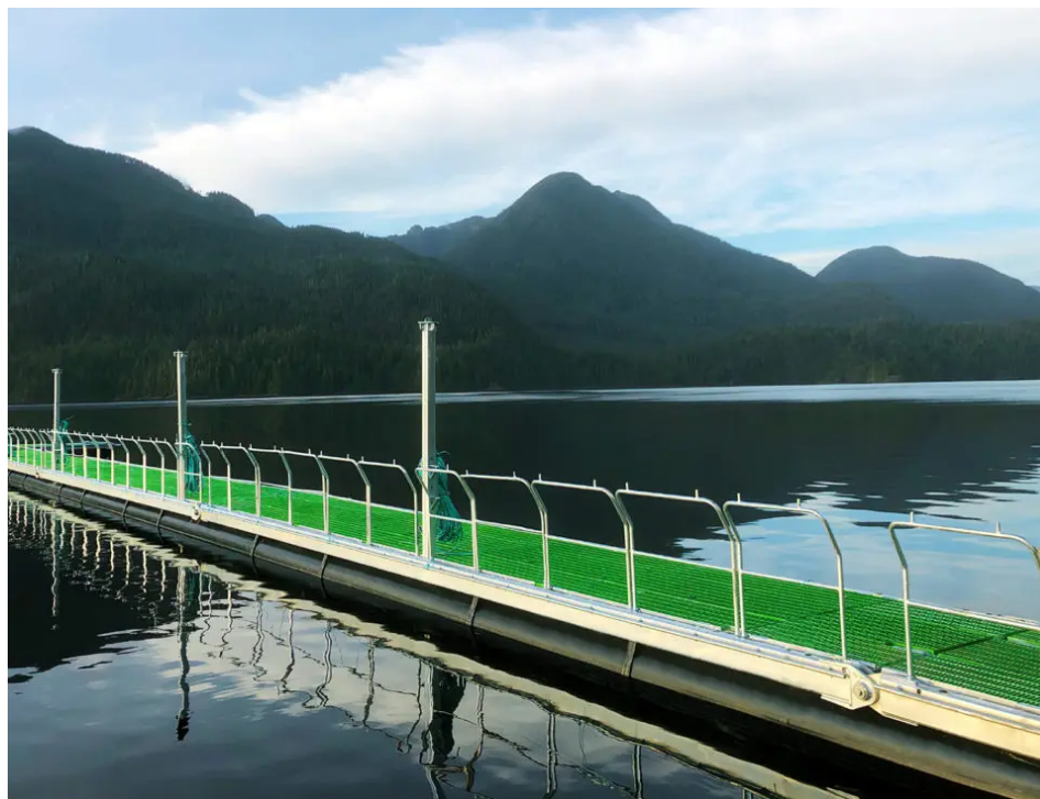
A sea-level view of the Trident Hybrid™ Steel Cage System structure.
