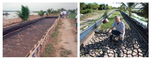
Sludge pens remove solids from dredge discharges before their release to the effluent canal.
