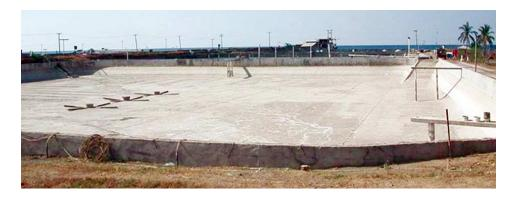
The most common pond construction in Indonesia uses concrete dikes and exposed bottom soils. This pond in northern Bali, which has a central drain and compressed air aeration, is fully lined with concrete. Photo courtesy of Tommy Chandra.
