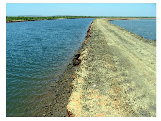
Settling basins retain sludge and remove suspended solids from water supplies. Proper construction can minimize erosion of the earthwork.
