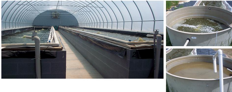
Wastewater from a shrimp raceway system was processed by two 500-L sequencing batch reactors at the Gulf Coast Research Laboratory.
