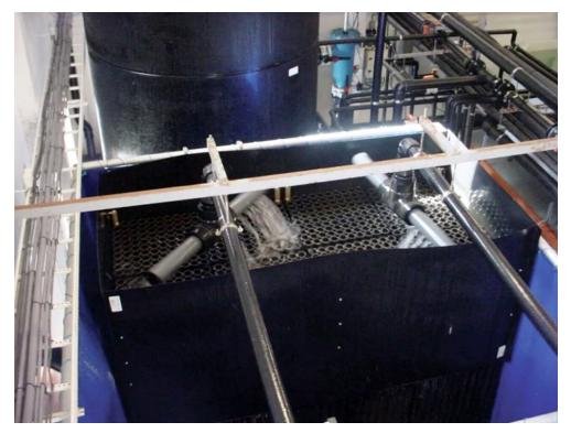
Trickling filters are simple, reliable filters that provide stable nitrification, water aeration and carbon dioxide degassing in one unit. In this example, water is sprayed over two trickling filters with rotating arms. Photo courtesy of AquaOptima, A.S.
