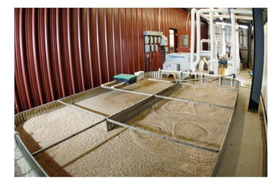
Moving bed reactors provide reliable, energy-efficient and compact biological filtration. Small plastic media is kept in motion by aeration or water movement within the reactors. Photo courtesy of North Carolina State University and The La Paz Group, LLC.
