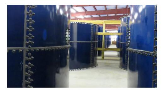
NaturalShrimp uses a gravity-flow system with vertically configured 10-foot tall tanks, which the company says results in more production per square foot. Courtesy photo.
