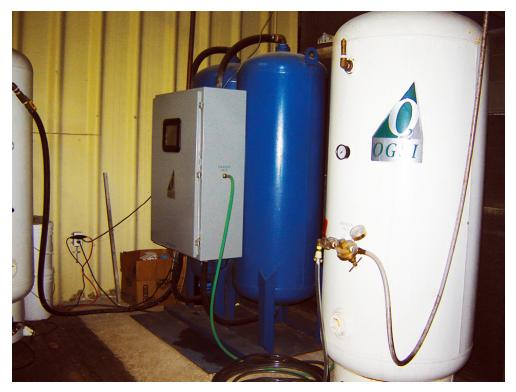
This oxygen generator and its oxygen storage cylinder employ highpressure swing adsorption to produce oxygen.
