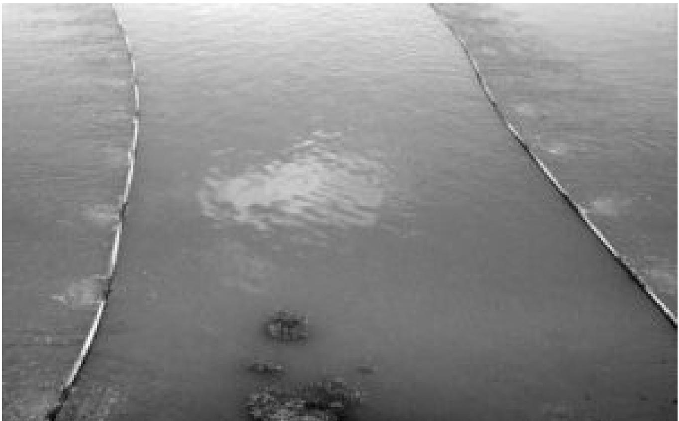
Diffused-air aeration systems release bubbles of air near pond bottoms to rise through the water column.
