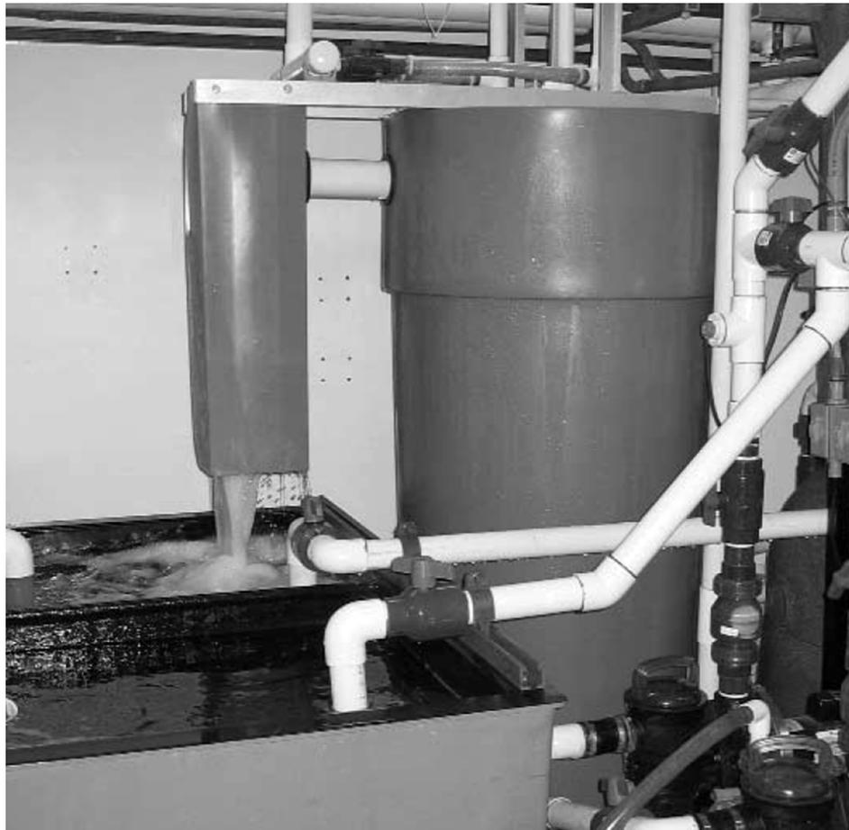
Fluidized-bed biofilter in operation. Photo courtesy of Aquaneering Inc.
