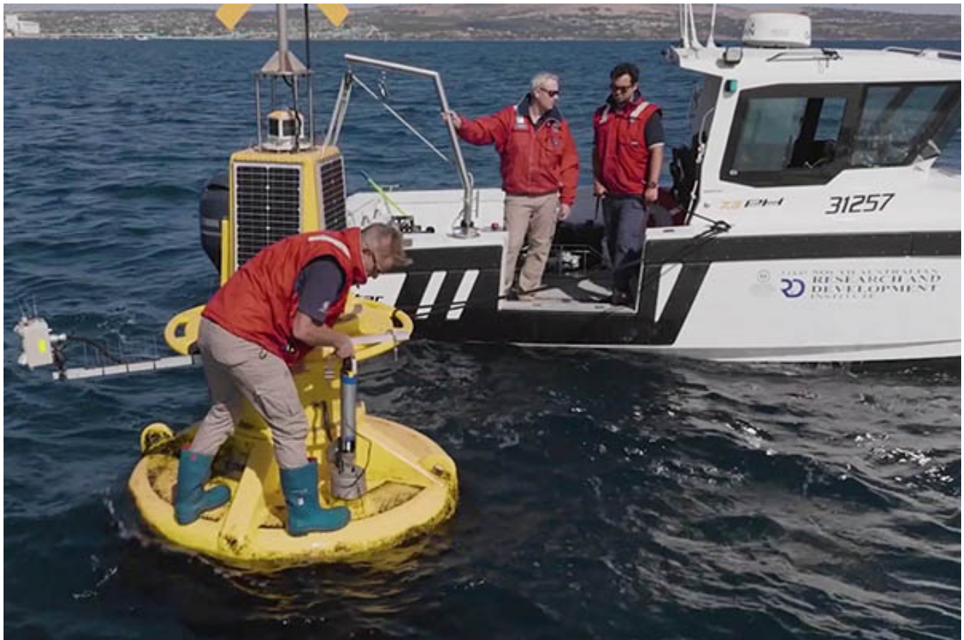
The SARDI research team replaced one of the water sensors on the AquaWatch buoy in the Spencer Gulf. Photo courtesy of CSIRO.
