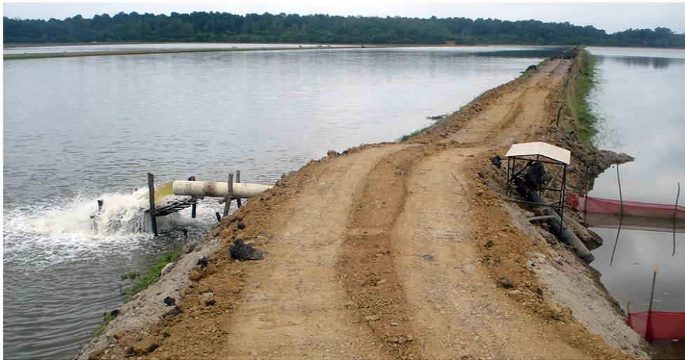
At retrofitted farms, water from ponds used as recirculation units is pumped across levees to production ponds.
