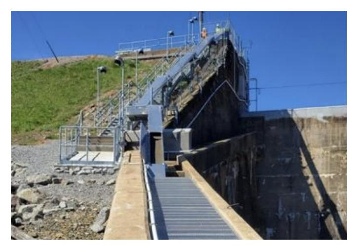
The permanent eelway (enclosed stainless steel structure) at Blewett Falls Dam is built into a retaining wall (the concrete structure with metal screening) on the southern bank of the Pee Dee River. As juvenile American eel approach the dam, they are attracted into the eelway entrance by favorable flows, and the scent of other eels in the holding tank at the top. Photo credit: Justin Dycus/Duke Energy.
