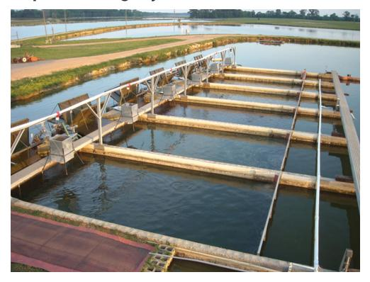
Paddlewheels on the upstream side of the raceways allowed frequent water exchange within the closed pond system.
