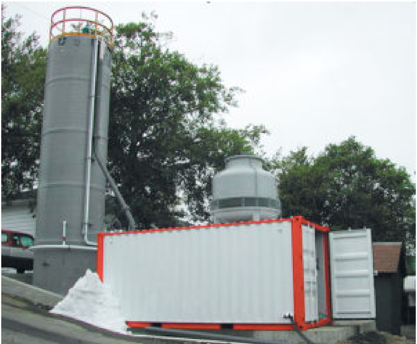
New self-contained mobile systems feature “containerized” ice slurry generation, pumping and controls.
