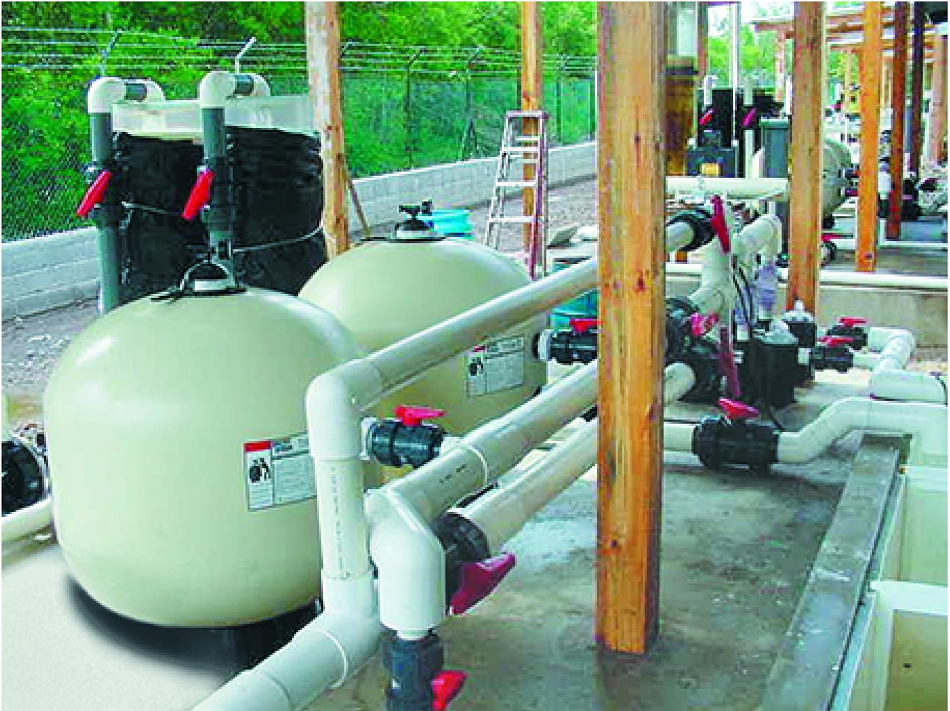
Rapid sand filters (foreground) mechanically filter waste in advance of the biodisc biofilter (background).
