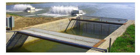
After treatment in the algal basin, water returns via sluiceway to the fishconfinement area. Aerators are typically run only at night.
