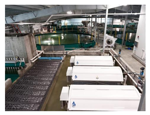
View of the water treatment area of Kuterra LLC, a commercial RAS facility near Port McNeill, BC, Canada. Note the array of 500-cubicmeter culture tanks in the background, and the fish pump and mobile grader station. Photo by J.R. Rardon.
