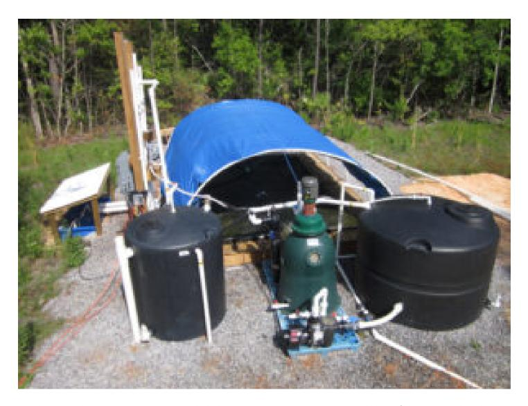
The secondary treatment system included a supernatant reservoir tank, polishing filter, activated carbon filter, ultraviolet treatment and tank aeration.
