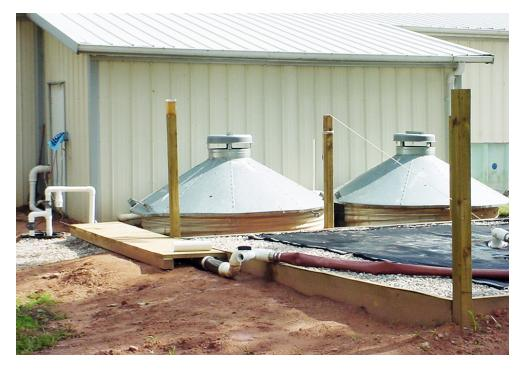
A geotextile bag (on left) rests on a rock-filled effluent containment system that collects the clarified effluent on a rubber liner and directs it to a clarified effluent sump. Recirculating aquaculture systems (RAS) have often been referred to as green and environmentally friendly technology. This is in fact true, as long as the effluents from these systems are dealt with adequately and responsibly.
