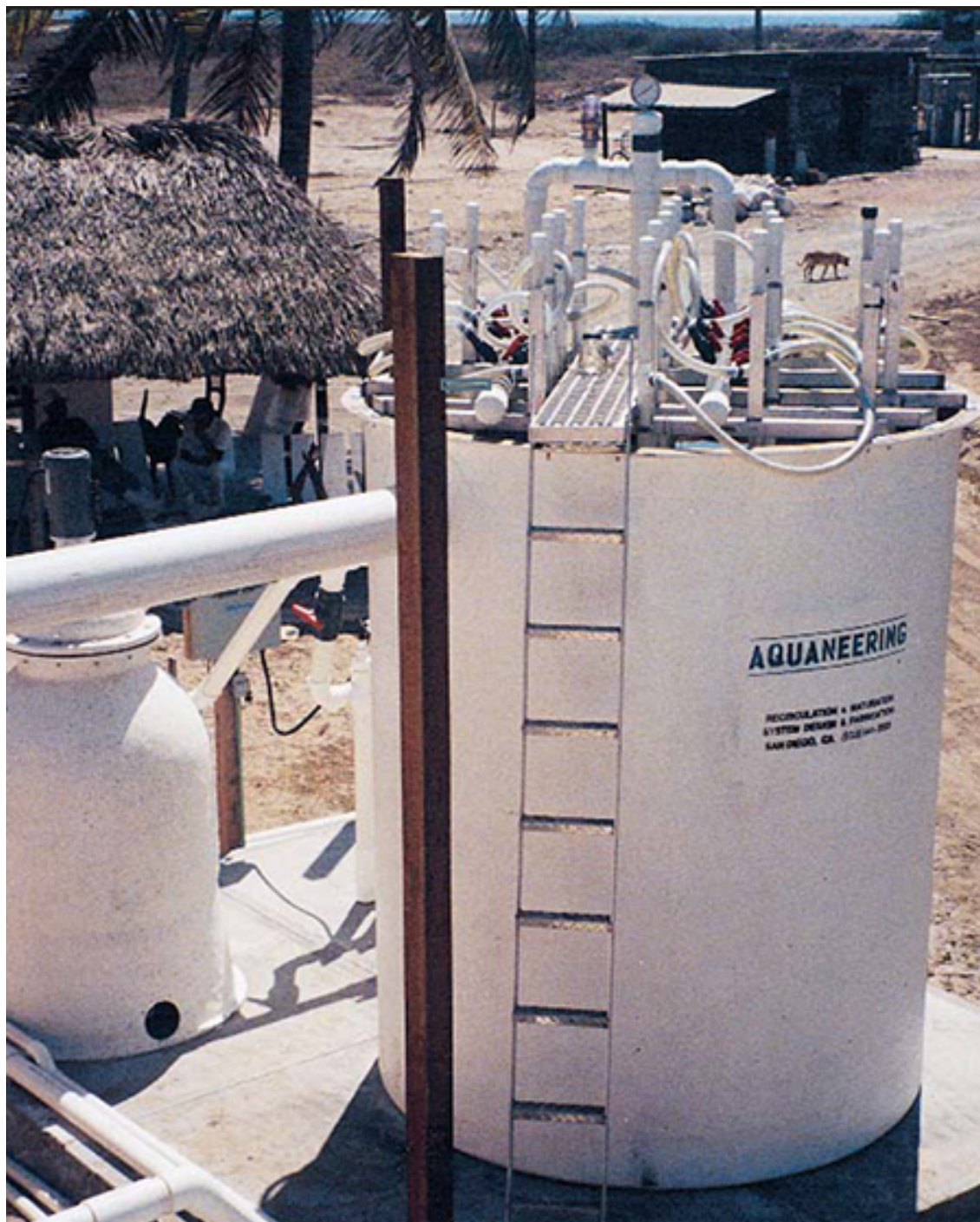
Fluidized bed biological filter with a flow rate of 15 liters/sec (200 gallons per minute).
