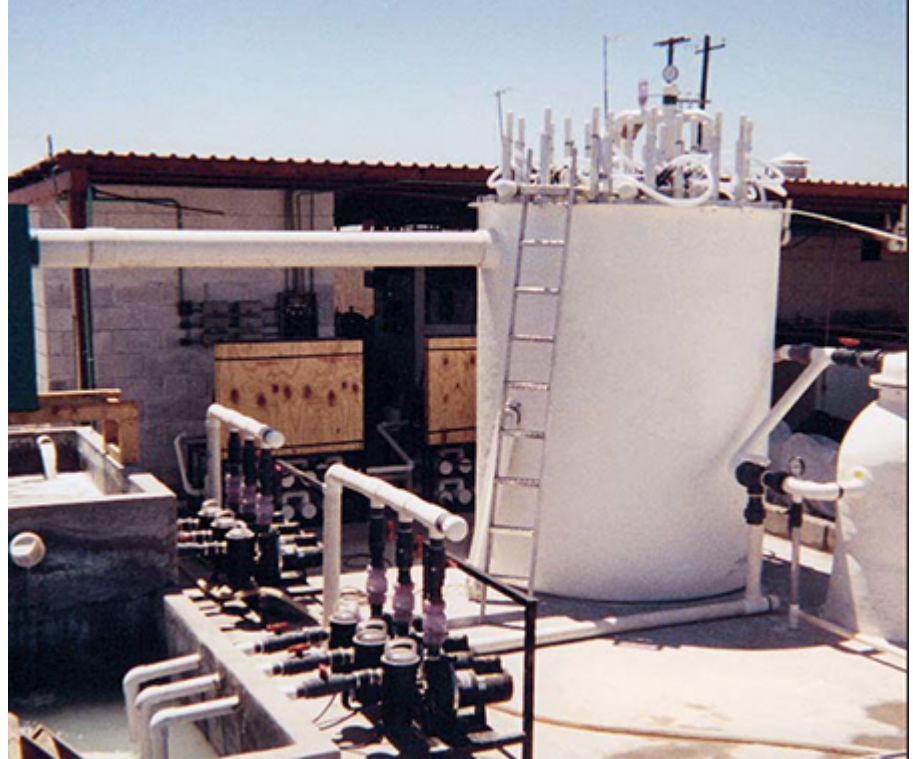
Complete fluidized bed filter system for shrimp maturation.
