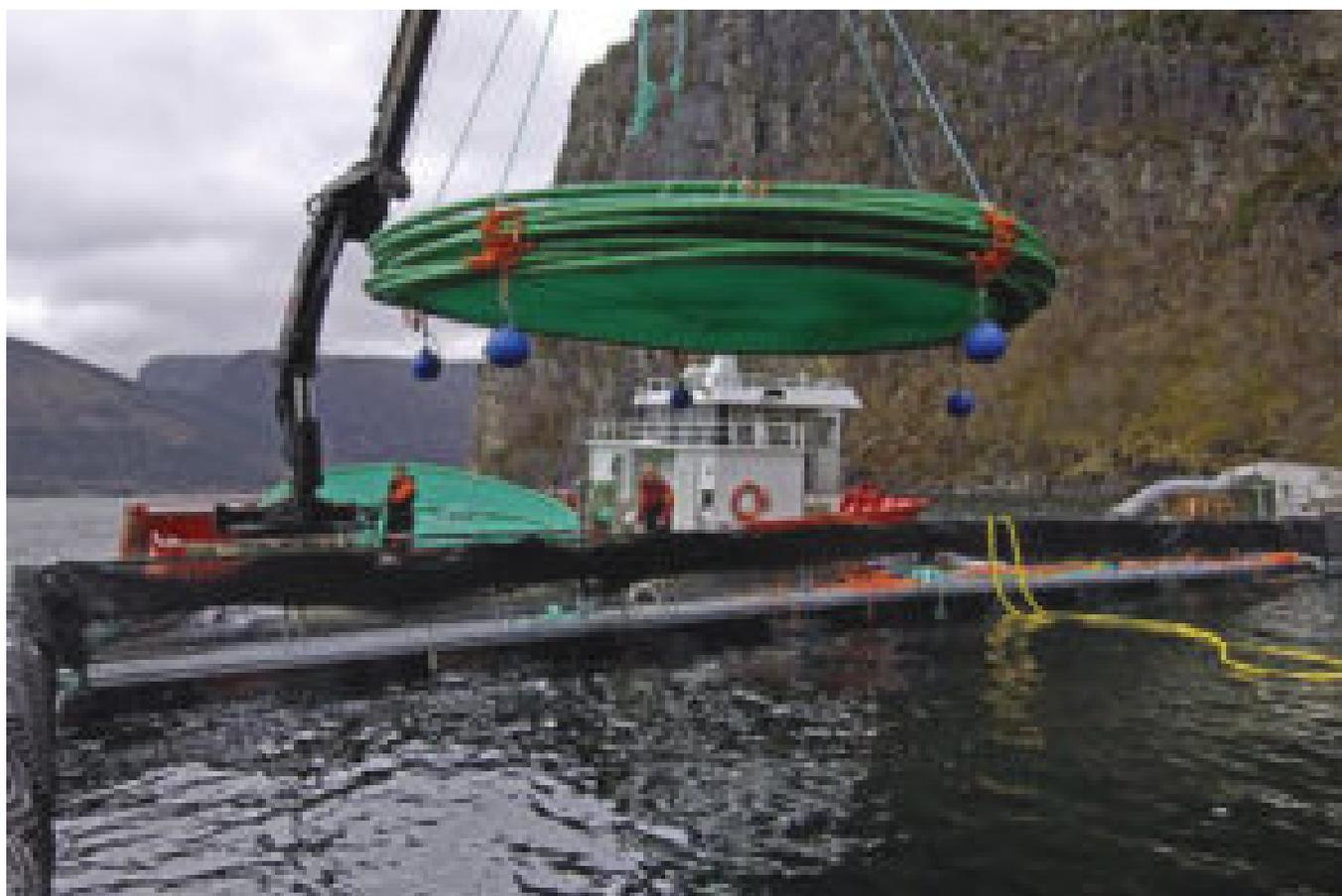
Multilevel stacked “decks” with net floors are lowered into larger net pens to provide living area for the halibut, which in nature spend much time lying on the ocean bottom.
