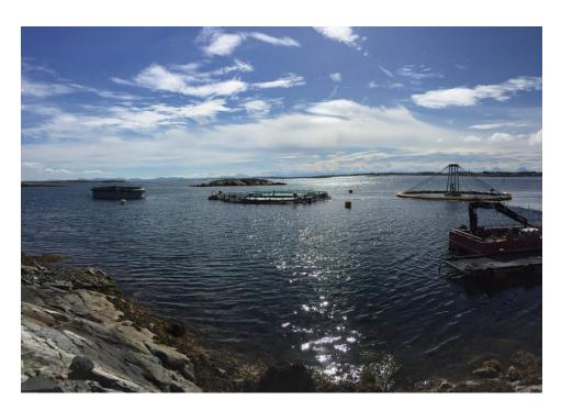
Three floating closed containment systems at Smøla/ Nekton Havbruk AS, i.e., from left to right: the "Salmon home #1" concrete tank (as it is being deployed), flexible floating semi-closed containment system, and Fiberglass AgriMarine tank. Photo by Jelena Kolarevic.
