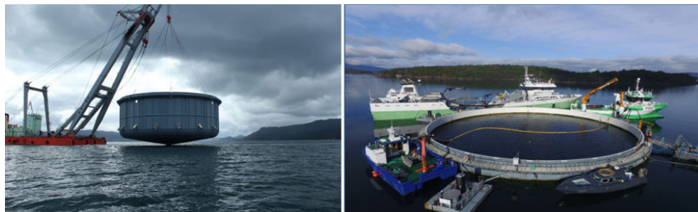
One of the closed containment floating systems of Marine Harvest Norway, owned by Aquafarm Equipment AS. Photo of Kjell Kleivland.
