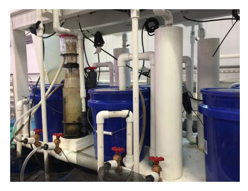
Filtration components such as foam fractionators and external biofilters may be used for RAS nursery production.
