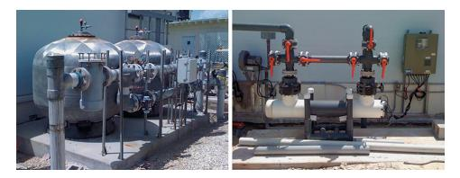
Current UMEH research on larval rearing and nursery stages uses filtered, ultraviolet-treated seawater.
