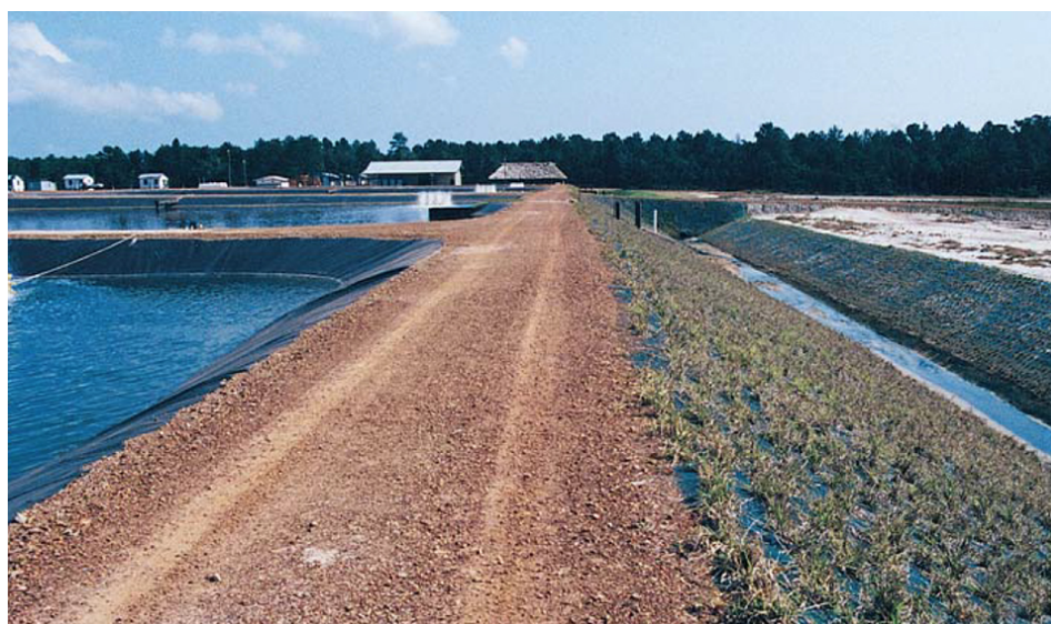
Pond levee showing plastic liner on left (wet) slope. Right (dry) slope is covered with fabric mesh and sprigged with grass to control erosion.
