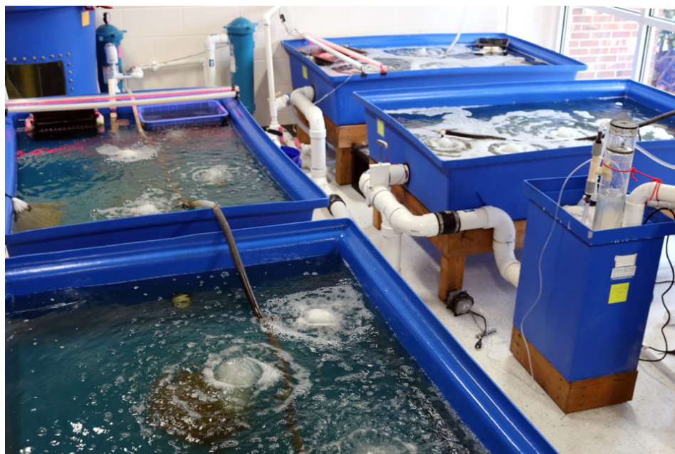
A look at Kepley BioSystems’ RAS set-up for horseshoe crab research.
