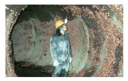
Mussels attach to and grow on the surfaces of power plant water intake pipes.
