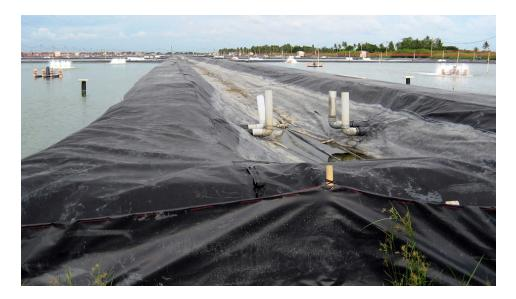
Liners increase biosecurity and stabilize dikes and supply canals.
