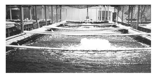
Floating vertical pump aerators supplement blowers and help keep solids in suspension.
