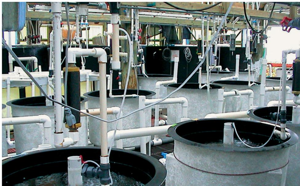
Changes to reduce bacteria levels in the research hatchery included improved system design, better management and the optimization of pipe sizes and reduction of by-passes and other regions where bacteria might accumulate.
