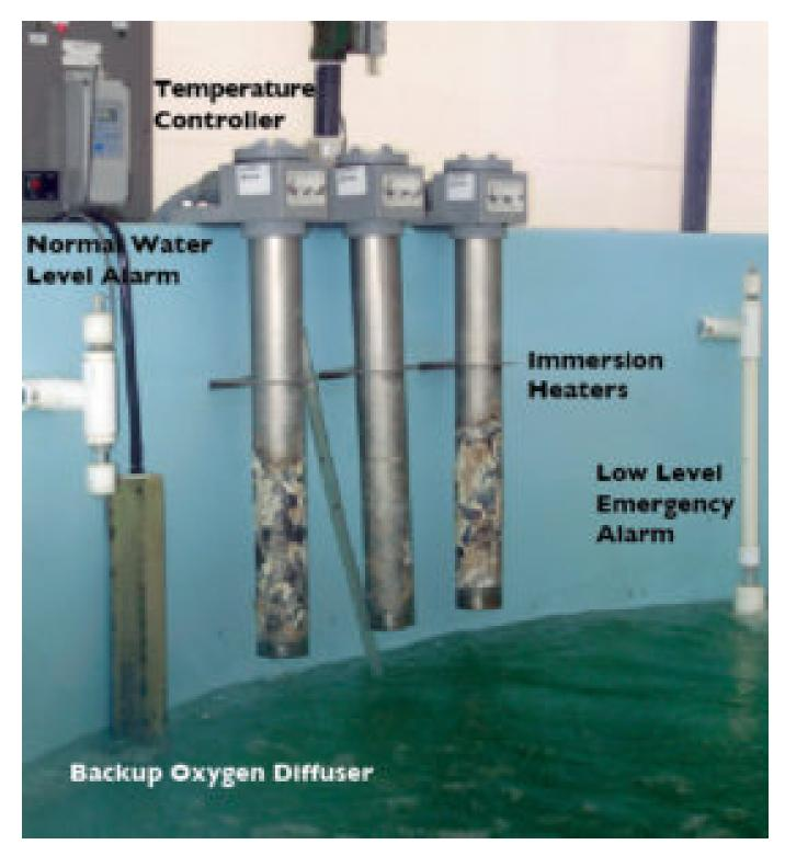
Float switches can monitor both low and high water levels, and act as a safety shutoff for submerged heaters in the event of a dramatic drop in tank water level.
