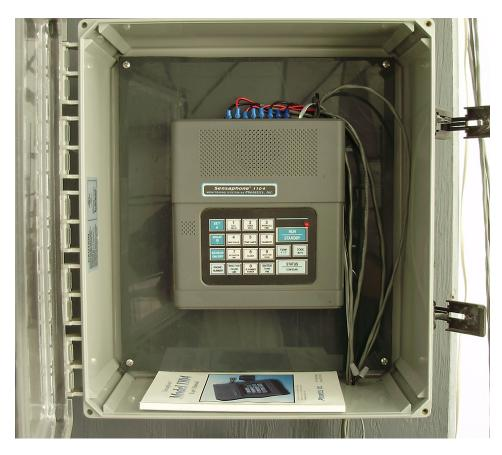
Phone dialers can immediately alert off-site staff to power loss and other system failures.
