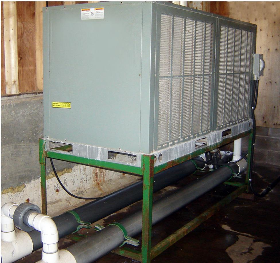
This high-efficiency, air-cooled water chiller for aquaculture has a coefficient of performance over 3.5.
